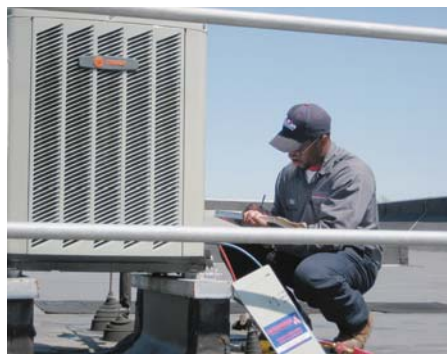
Technician Rich Britt...Maintenance pays!
