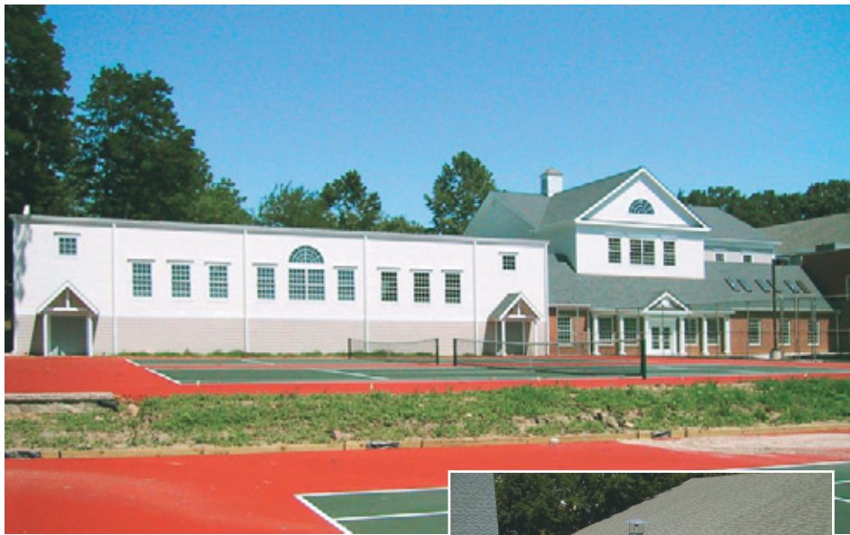
Above & at right: The new Moorestown Friends School Field House Architect: McGillin Architecture, Bala Cynwyd, Pa. Mechanical Engineer: Edward Fox, Bala Cynwyd, Pa. CM: E. Allen Reeves, Abington, Pa.
